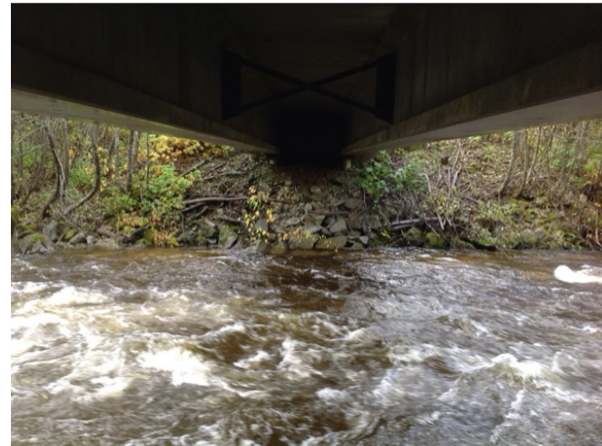
Left Bank Abutment when facing downstream
