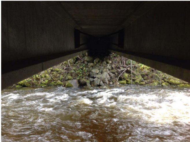
Right Bank Abutment when facing downstream
